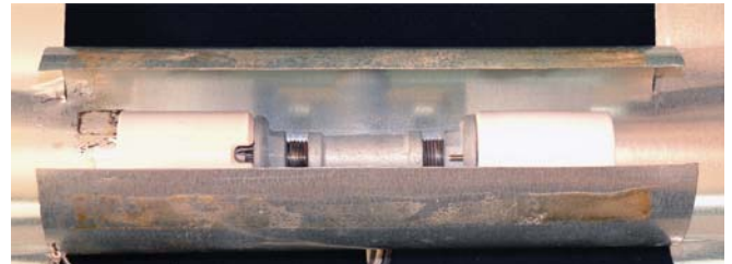
4. Mogul bases installed.
