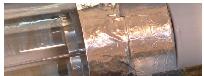
7. Tape with 2 inch FOIL tape insert to 1 inch
