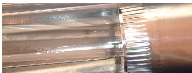
10. Attach a duct connector kit to each end.
